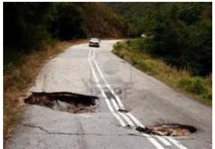
Only 17 % of the roads in Ghana have asphalt. Here is one of them but with some large potholes - unfortunately very common.
